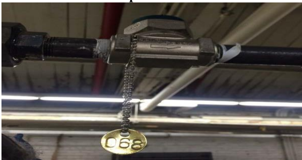
FIGURE 4: Steam Trap
